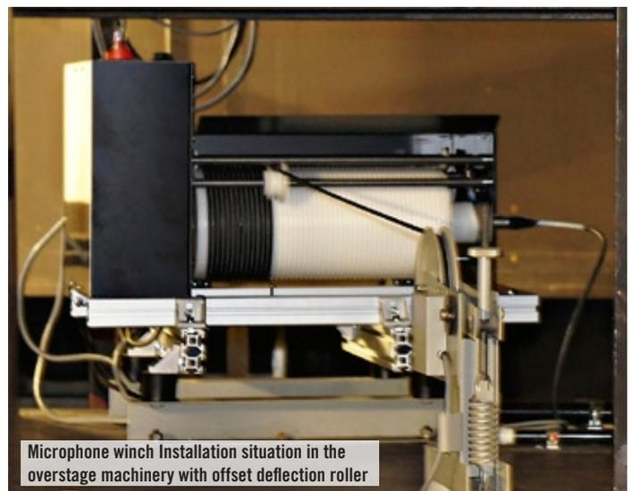
Microphone winch installation situation in the overstage machinery with offset deflection roller
